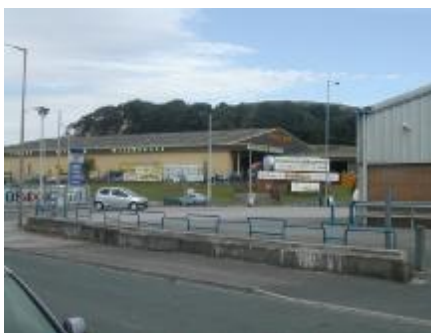
Canal Road: dominated by functional townscape character
